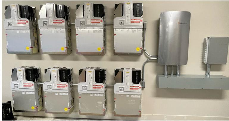
**Figure 1: Backup system - IQ Battery 5P (without cover)**
